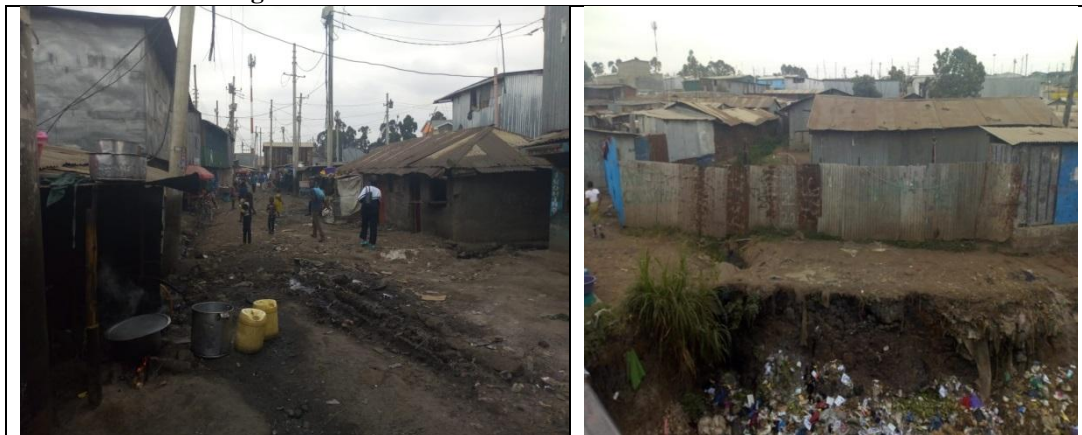
Figure 1: Shows Structures in Kiambiu Settlement.
